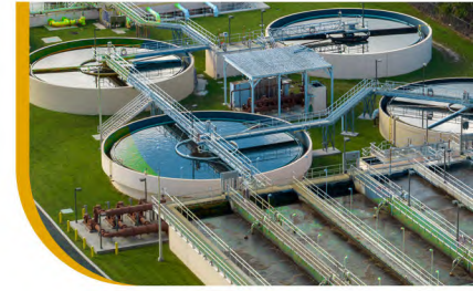
Sewage Treatment Plant
