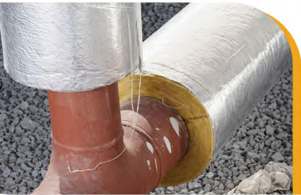
Pre Clad Insulation
